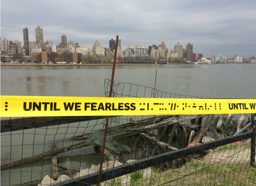
Above: Site excavation with Bobcat for Meg Webster's Concave Room for Bees Below: Installation of Marked Space by Brendan Fernandes
